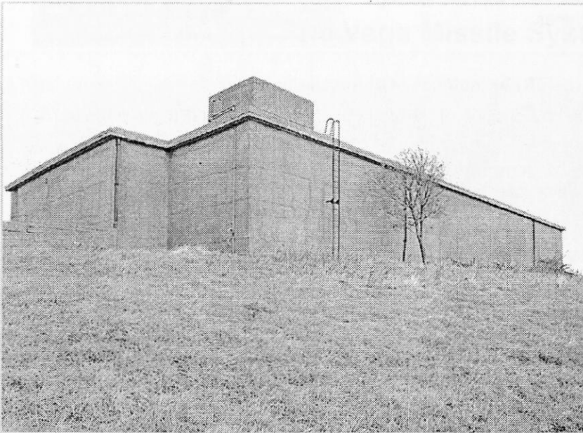
R6 Operations Block © Nick Catford
